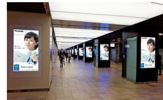
70-inch full high-definition LCD displays are mounted on the columns in the passageway leading to the ticket gates, which are slightly thinner.
